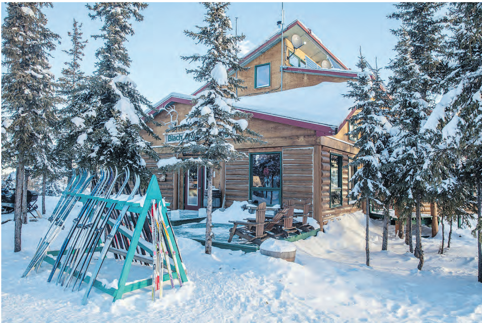
Power from solar panels, a wind turbine, a generator and five sets of batteries make Blachford Lake Lodge self-sufficient.
