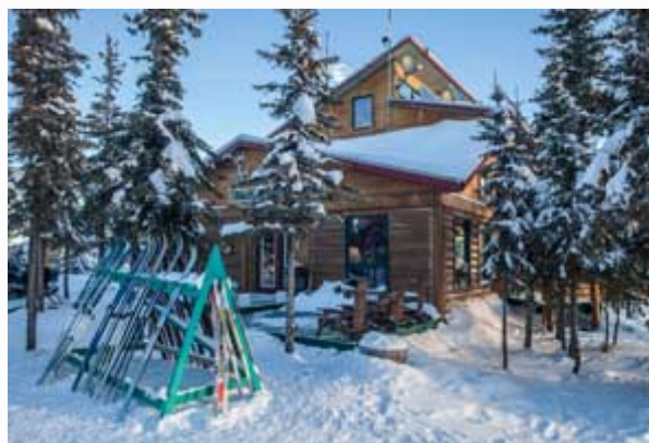
Power from solar panels, a wind turbine, five sets of batteries and a generator makes the lodge self-sufficient.
