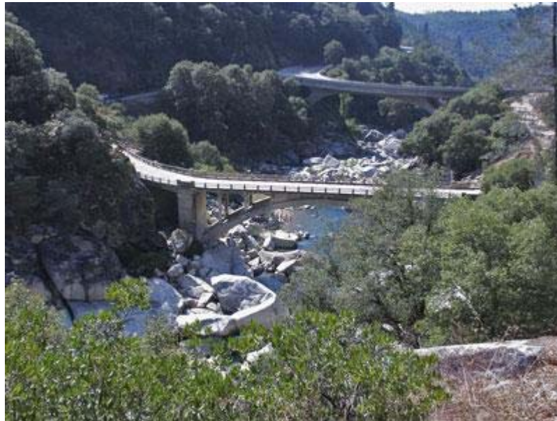
The South Yuba River with the old Highway 49 bridge (foot traffic only) in the foreground and the new bridge. (ColorWorld / Steve Haggerty)
